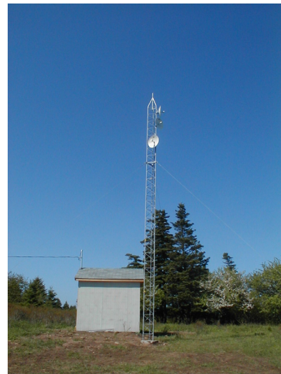
Fig. 8. MEPS Shore Station with Antenna Mast
